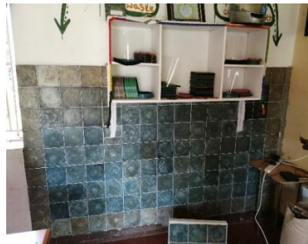
Image 13. Wall tiles representing 650 recycled soda and water plastic bottles at TakaTaka Plastics office in Gulu, 21.5.2021, a.p.
